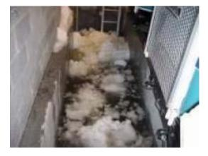
The dumping of ice resurfacer shavings outdoors would seem to be the simplest solution but there are also some risks, issues and energy efficiencies to be considered. Every time the ice resurfacer leaves the building the equipment door will be left wide open. During cold months, the room will need to be rewarmed while warmer seasons will allow moist air to enter the building and if not controlled will impact refrigeration, dehumidification and ice conditions.
