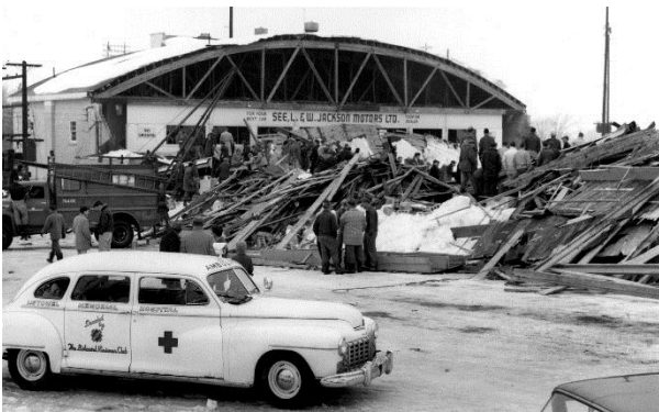
Listowel Arena Collapse, 1959 Killing 8 People
