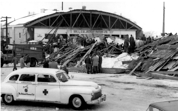
Listowel Arena Collapse, 1959 Killing 8 People
